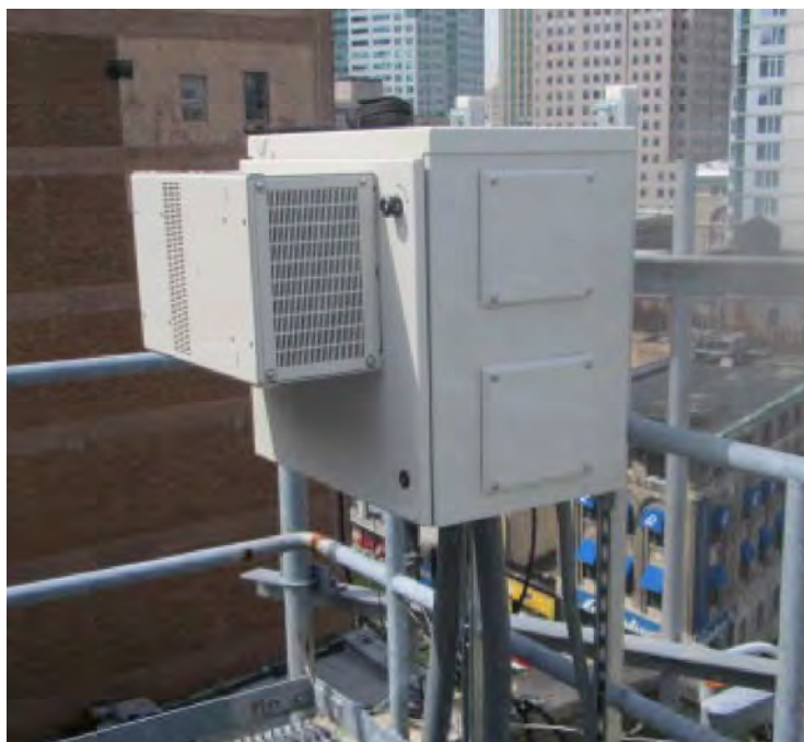
EMERSON NETXTEND COMPACT 2416 FIBER CABINET DIMENSIONS: 24.0"H x 24.0"W x 25.2"D WEIGHT: 64 lbs QUANTITY: TOTAL OF 1
