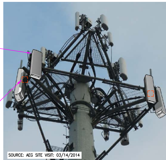
2 PROPOSED ANTENNA MOUNT TYP. A-3 N.T.S.
