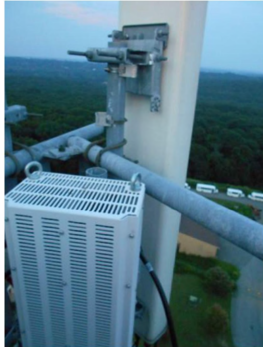
Photos of Verizon's typical existing equipment and mounts at 142'.
