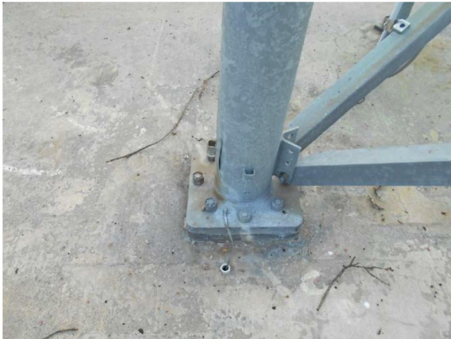
Photos of typical existing base foundation.
