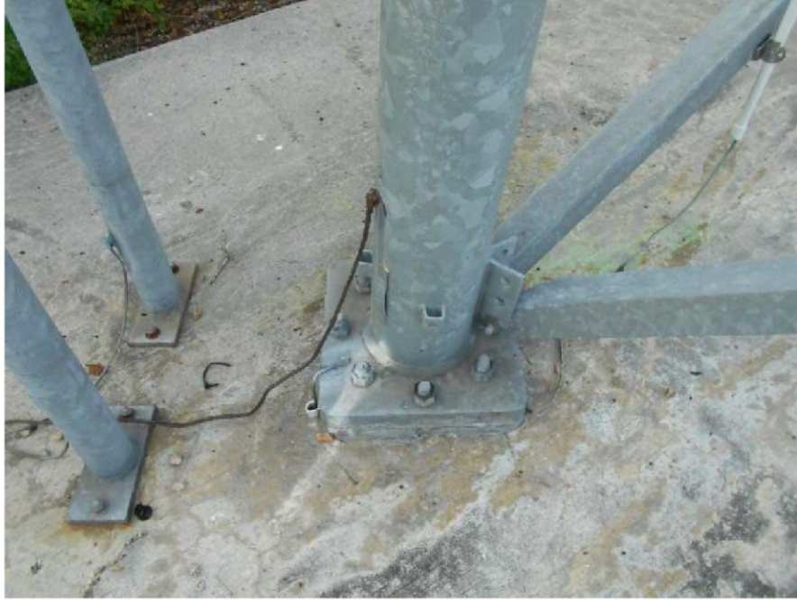
Additional photo of typical existing base foundation.
