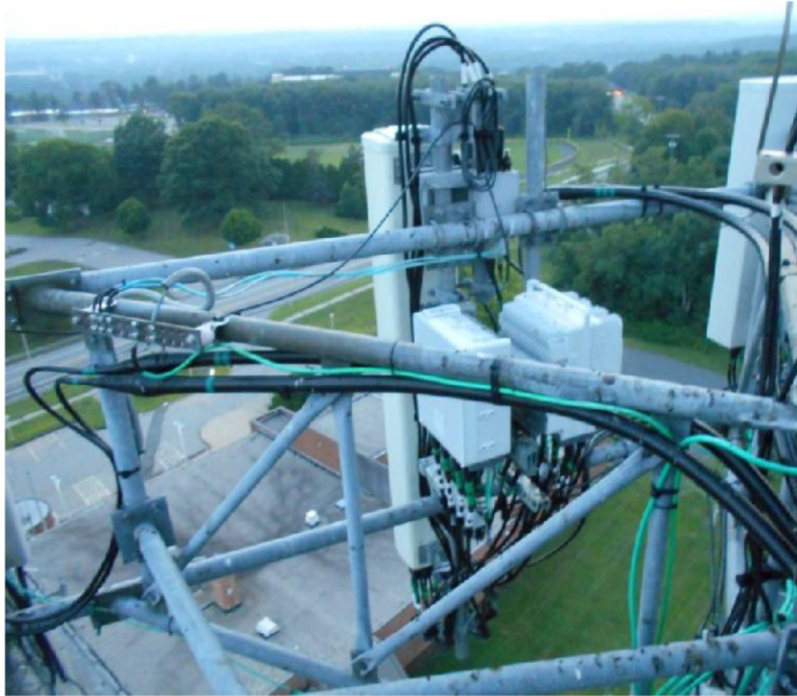
Photos of AT&T's typical existing equipment and mounts at 131'.
