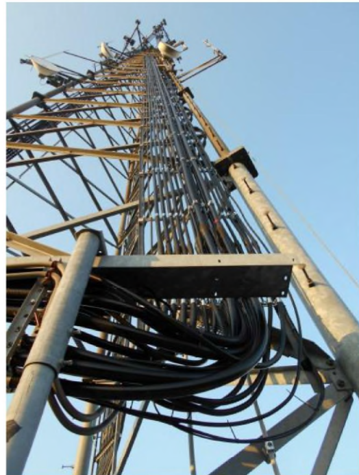
Photos of existing waveguide ladders on tower.
