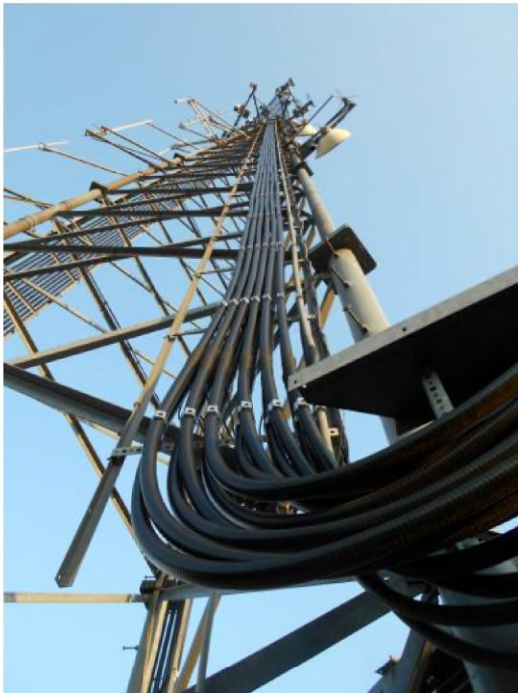
Photos of existing waveguide ladders on tower.
