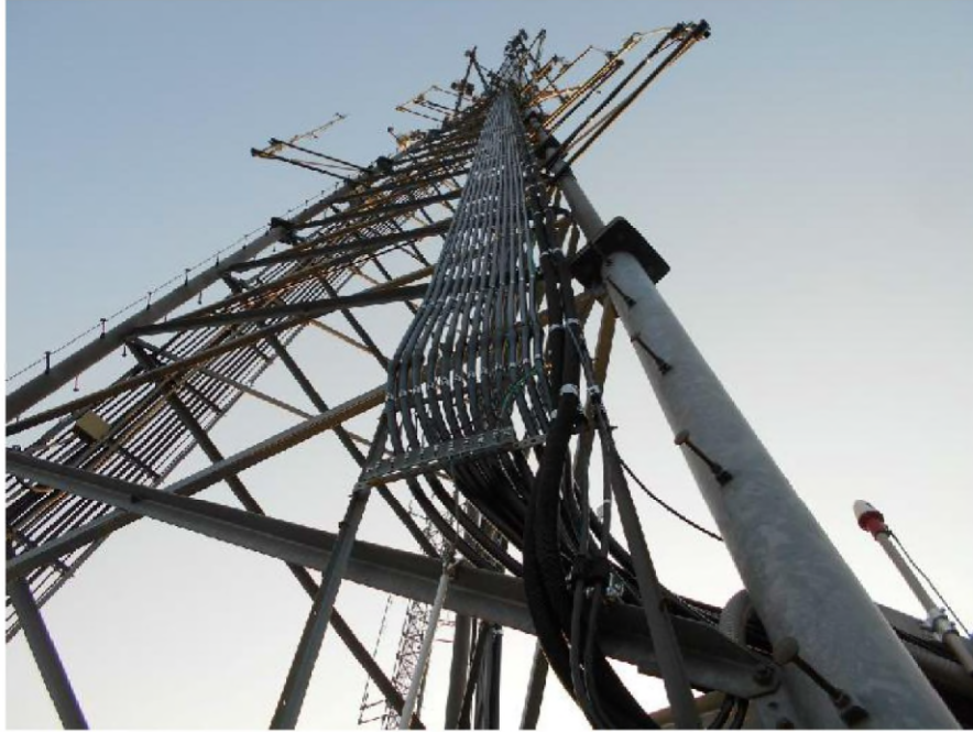
Photos of existing waveguide ladders on tower.
