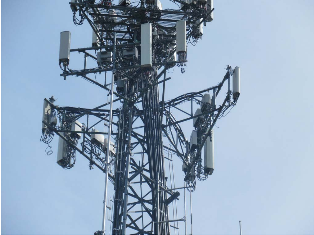
Photo 1: Photo illustrating the Tower with Appurtenances shown.
