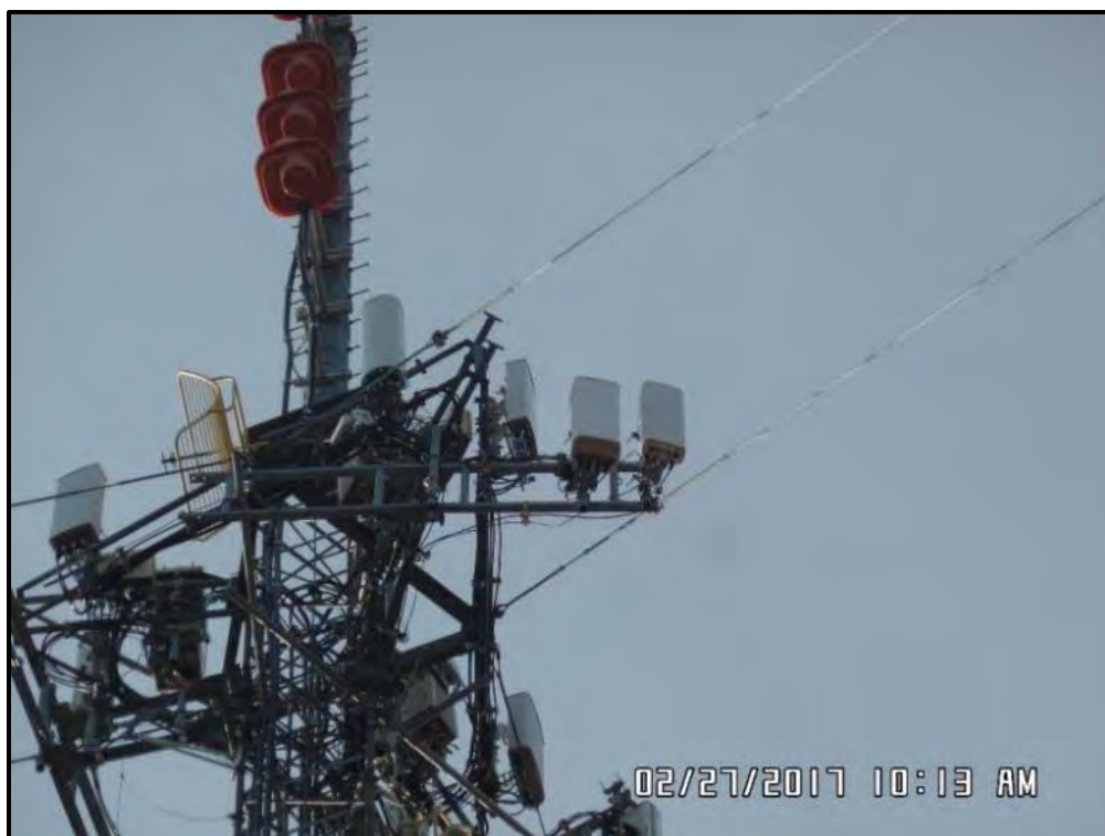
Gamma Sector Mount. Note antennas must be redistributed in mount face
