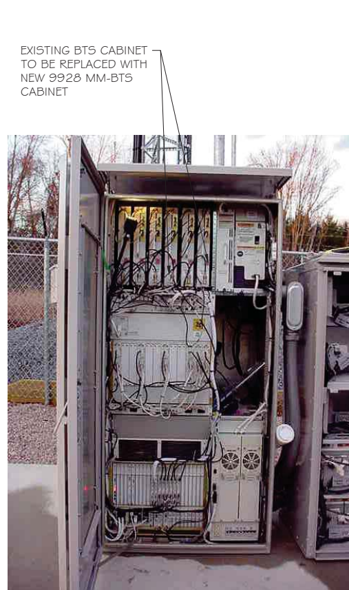
EXISTING MMBS CABINET SCALE: NTS
