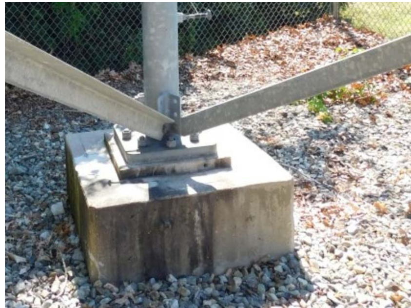
TOWER BASE LEG FOUNDATION PHOTO
