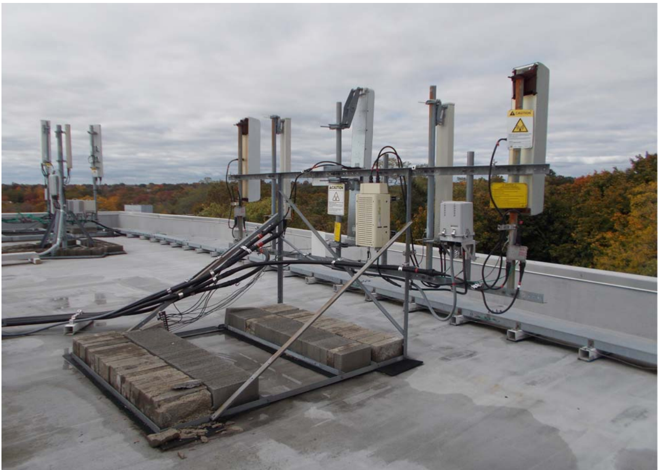
Existing Alpha Sector Ballast Frame
