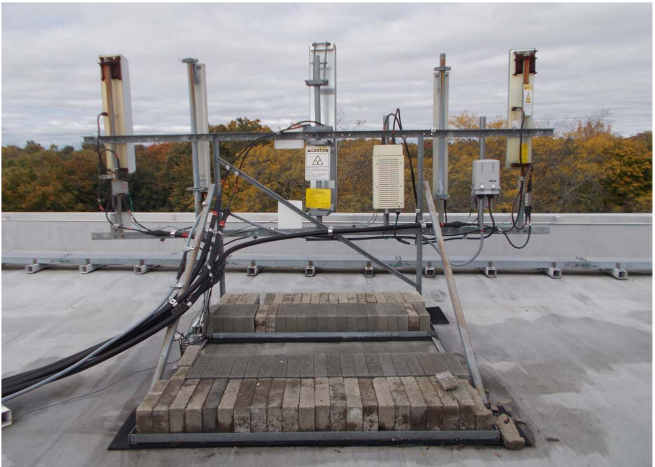
Existing Alpha Sector Ballast Frame
