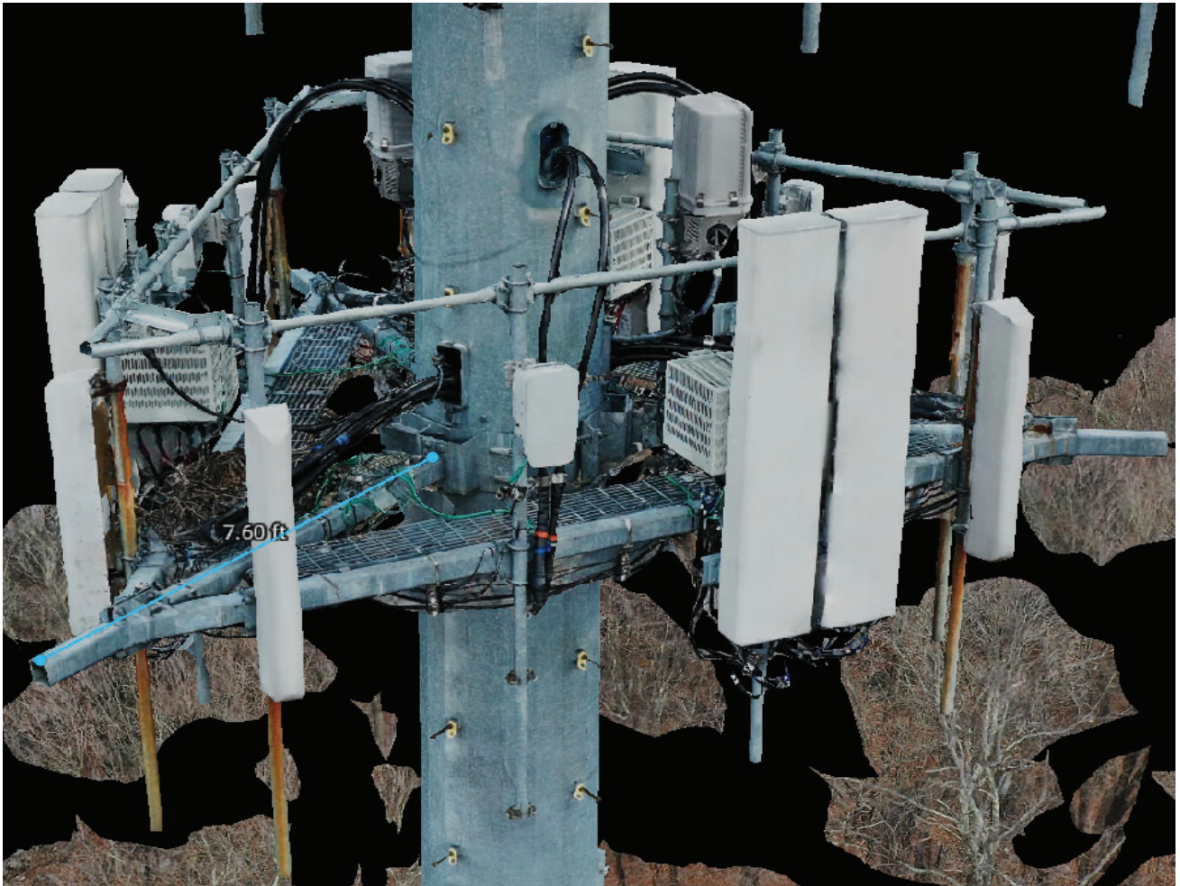
Image#9: Length of the standoff arms for T-arms and length of the inner bracings for platform (All sectors have same dimensions)
