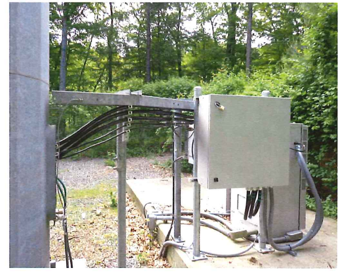
4 EXIST FIBER DISTRIBUTION BOX SCALE: NTS
