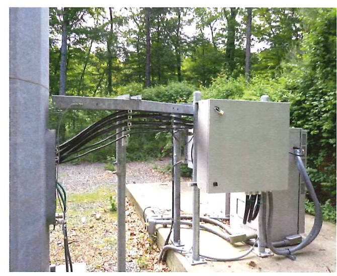
4 EXIST FIBER DISTRIBUTION BOX SCALE: NTS
