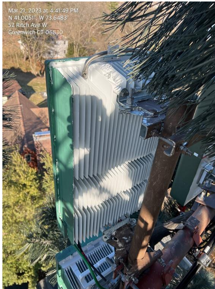
Photo - 2: Installation of proposed antennas in position 3
