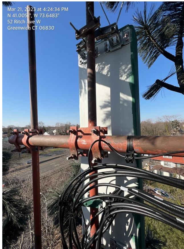
Photo - 1: Installation of proposed antenna in Position 2
