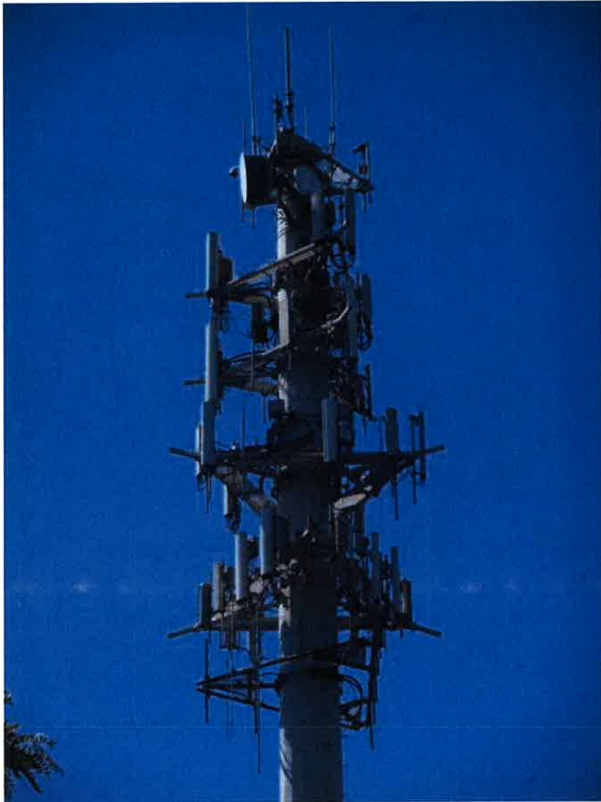
Photo 1: Photo illustrating the monopole with Appurtenances shown.
