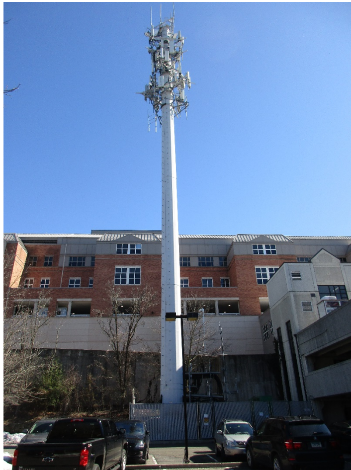
Figure 1: View of ES-158 Greenwich Hospital
