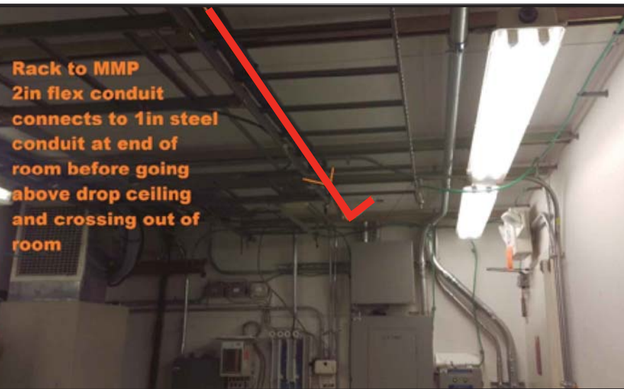
CONDUIT RUN FROM EQUIPMENT ROOM TO STAIRWELL
