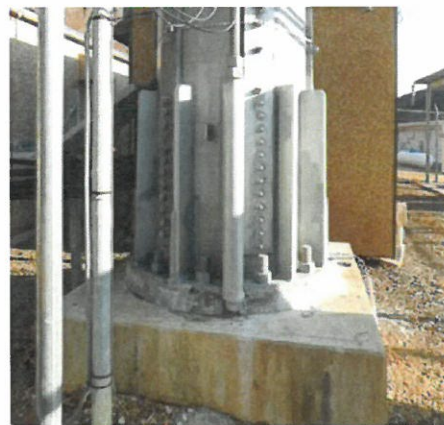
BOLT ON SAFETY CLIMB BRACKET INSTALLATION
