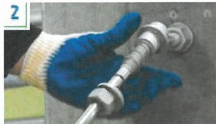
2 Remove the nut, the face washer and the spring shear sleeve and slide along the handle of the tool.
