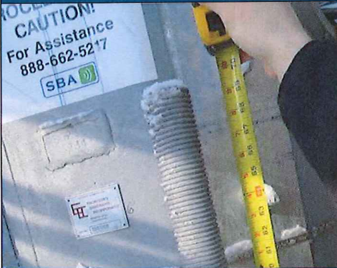
PH#11 Installation of Modification – New Anchor Rod Hole Depth Verification
