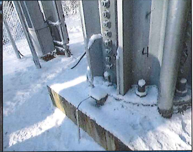
PH#12 Installation of Modification – New Anchor Rod Hole Depth Verification
