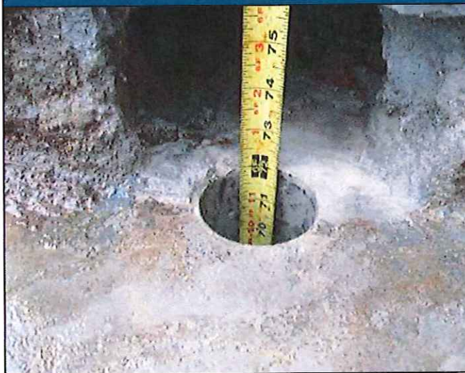
PH#11 Installation of Modification – New Anchor Rod Hole Depth Verification
