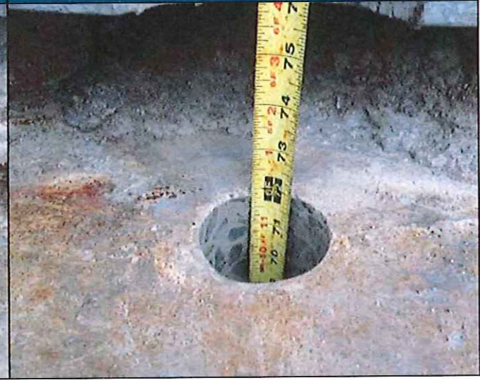
PH#12 Installation of Modification – New Anchor Rod Hole Depth Verification
