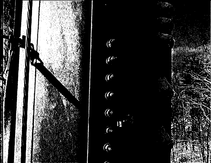
PH#16 Installation of Modification – Verification of Flat Plate Size
