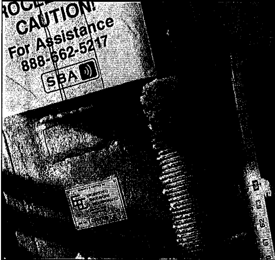
PH#11 Installation of Modification – New Anchor Rod Hole Depth Verification
