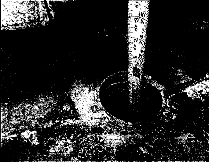
PH#15 Installation of Modification – Splice Weld Height Verification
