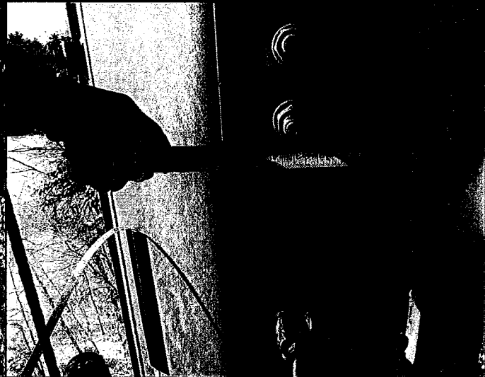
PH#20 Installation of Modification – Verification of Ajax Bolt Spacing
