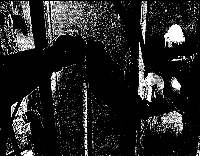
PH#15 Installation of Modification – Splice Weld Height Verification
