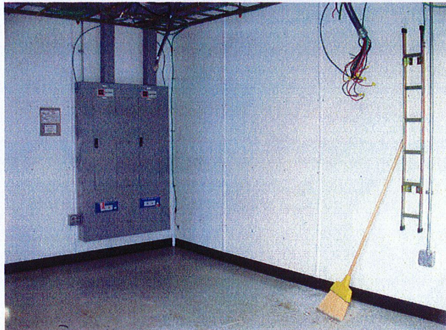
INSIDE AT&T FORMER SHELTER (EQUIPMENT REMOVED)
