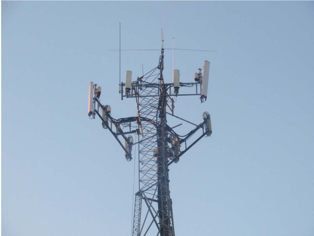
Photo 1: Photo illustrating the Tower with Appurtenances shown.
