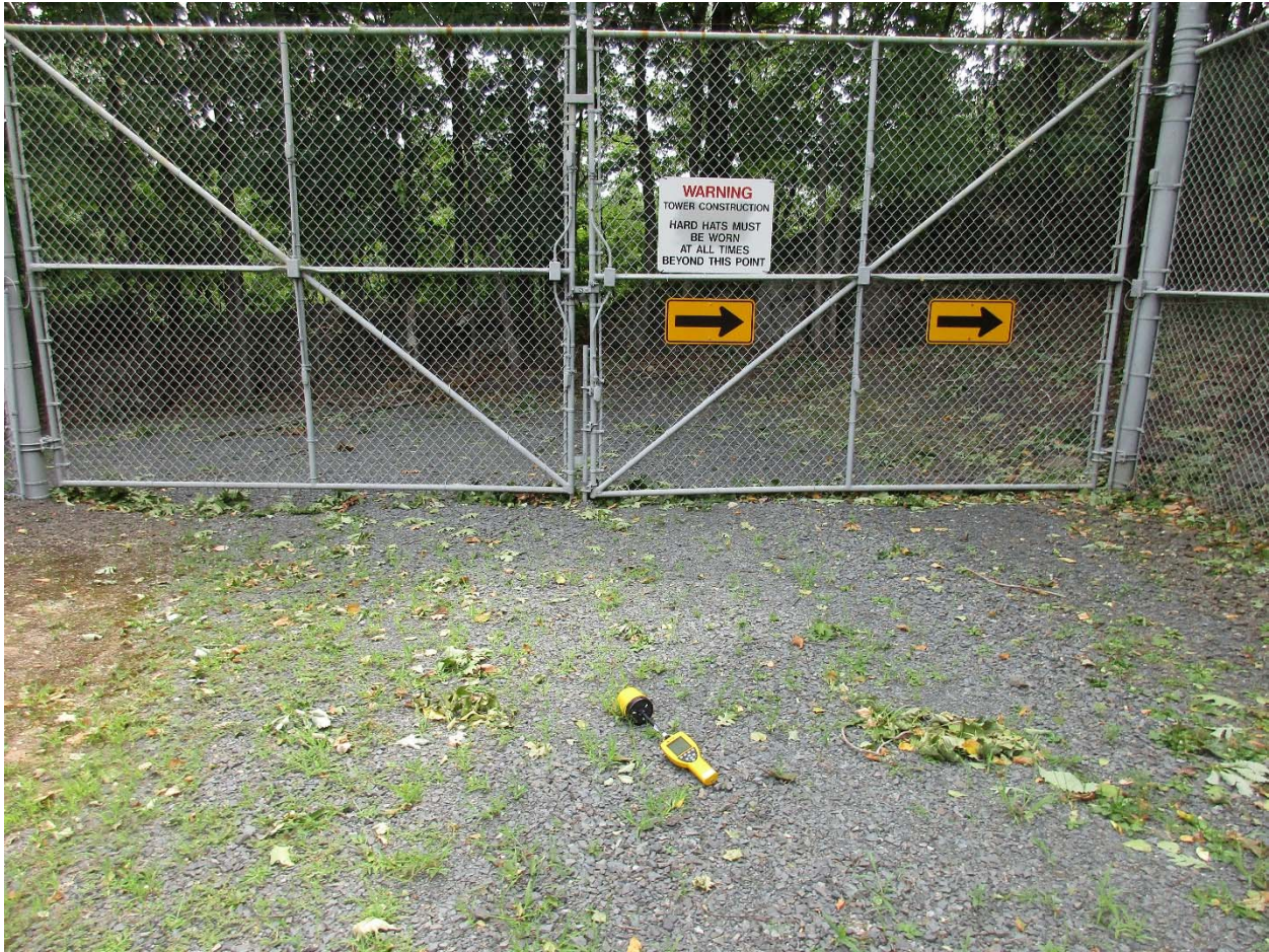
Figure 10: Measurement Location 7 (Southeast Gate)
