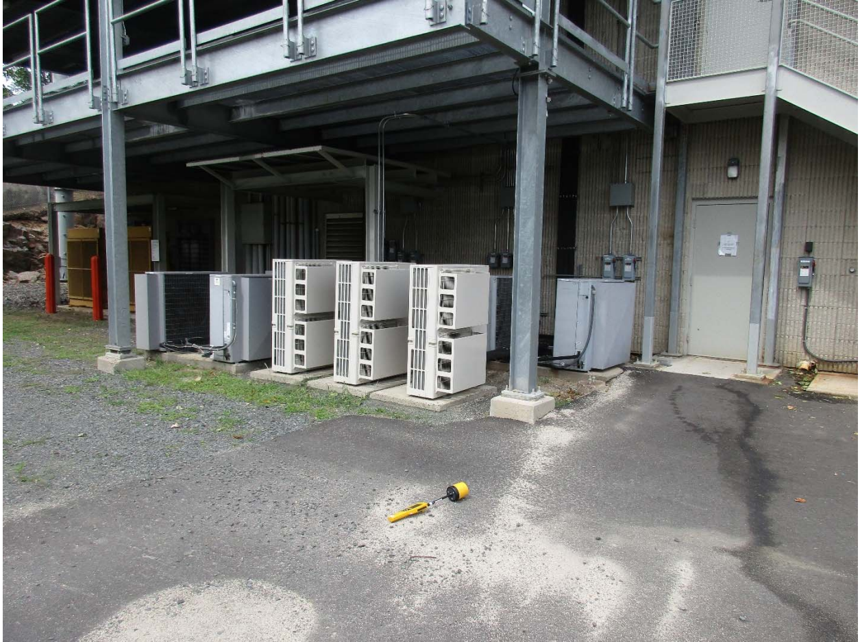
Figure 12: Measurement Location 9 (East of Building)
