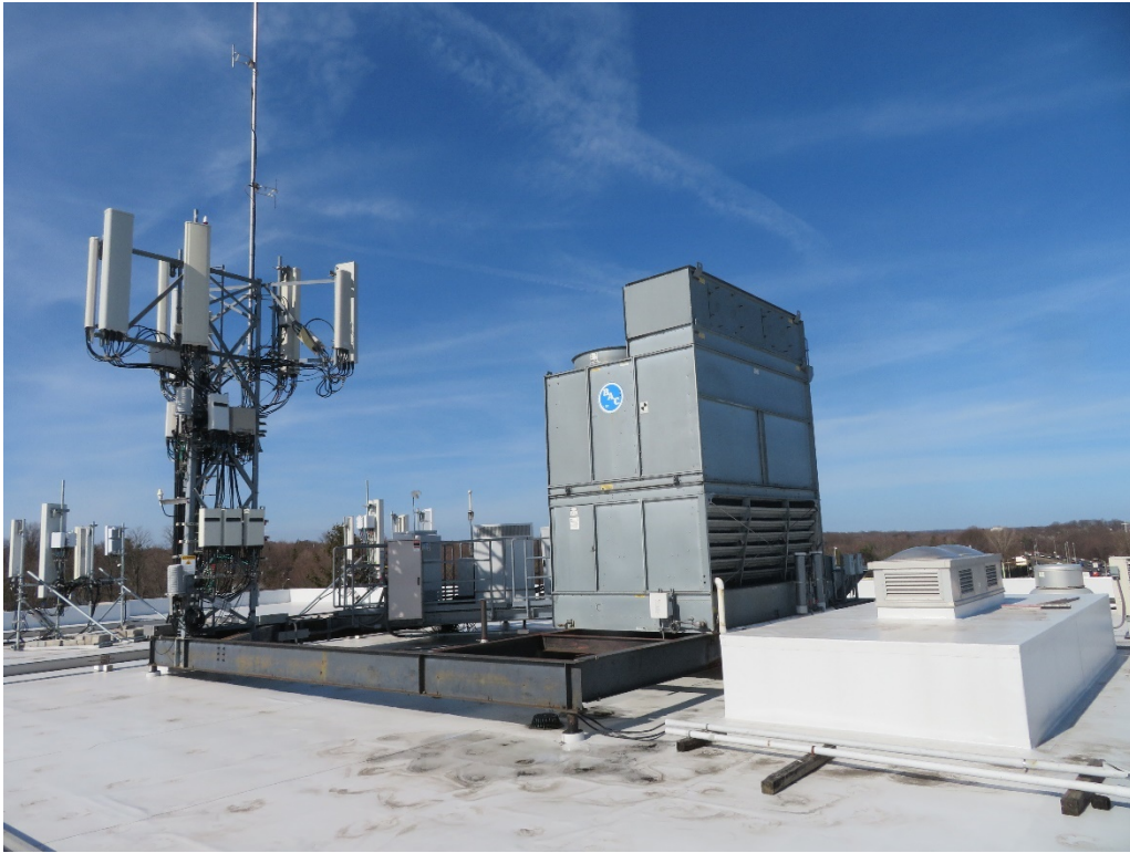
Photo 1: Sample photo illustrating the existing tower and steel platform.
