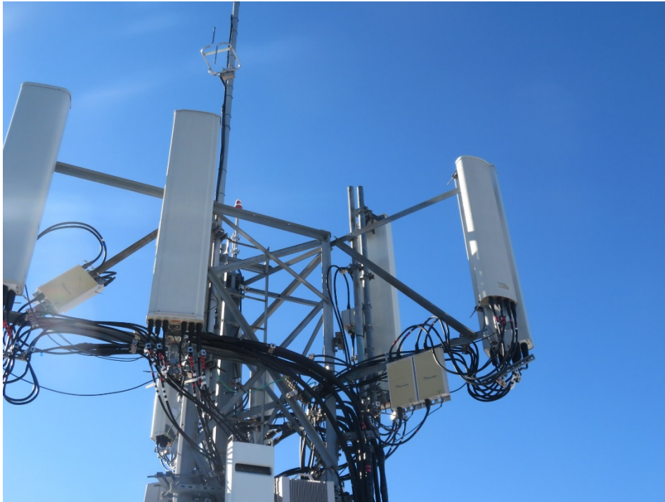
Photo 1: Photo illustrating the Tower with Appurtenances shown.
