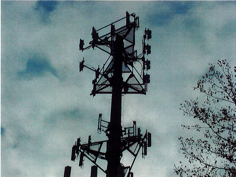
AT&T Antennas before removal
