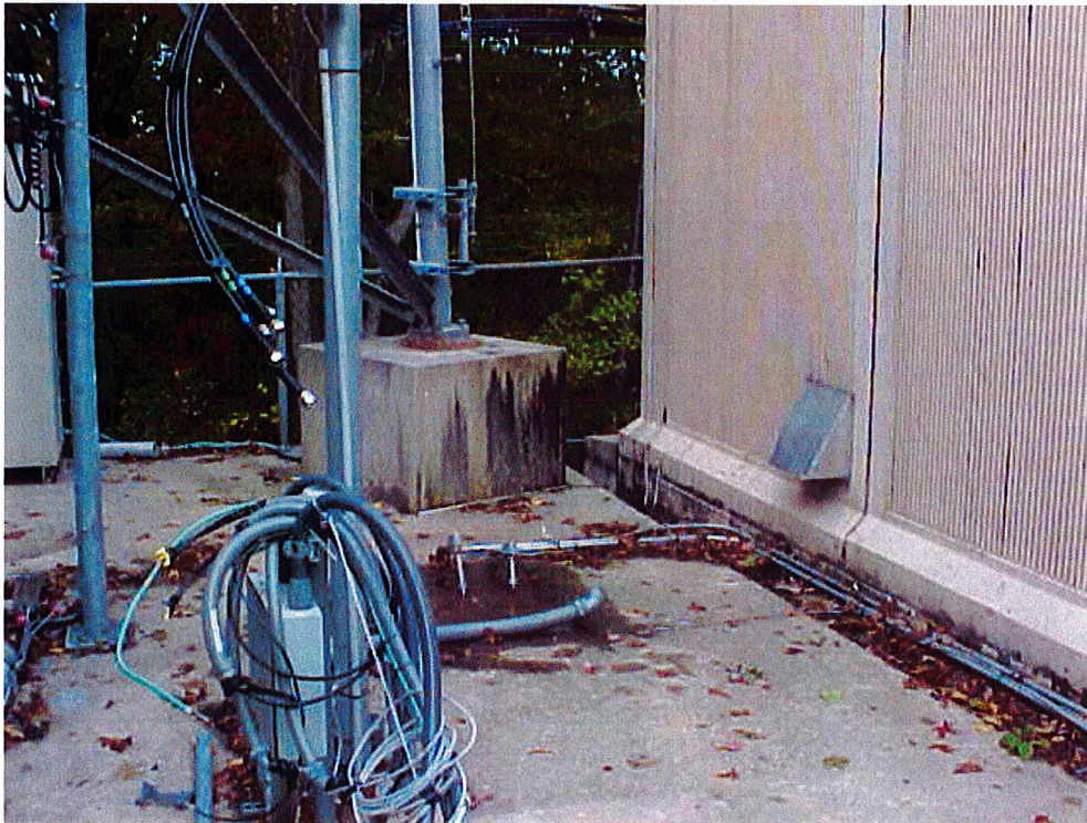
After base station removal
