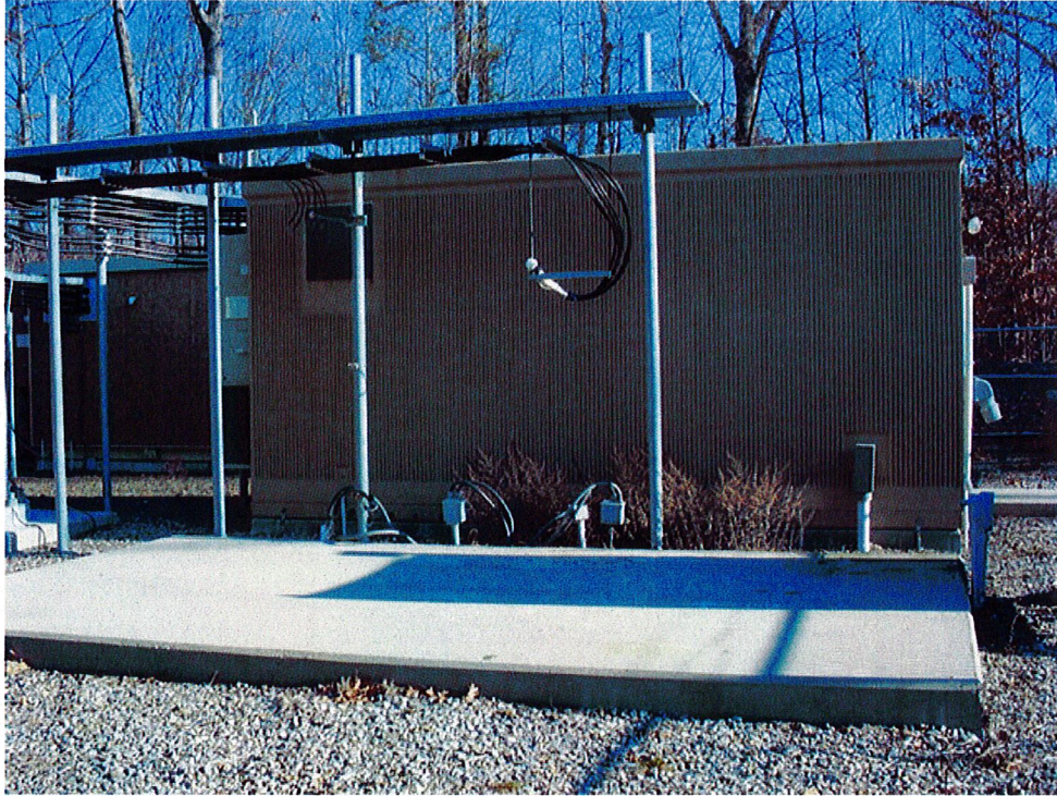
Before cable removal
