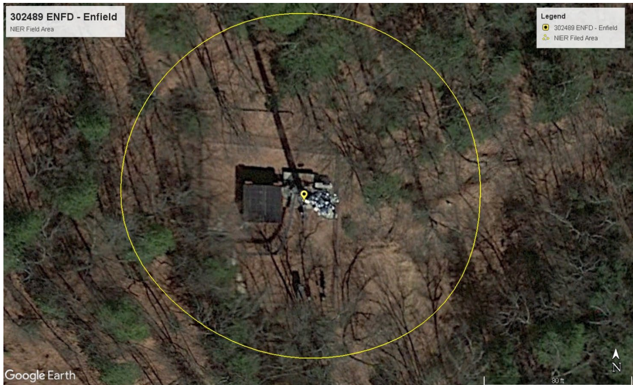
Aerial View of Site
