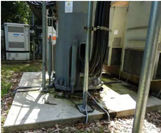
TOWER BASE/FOUNDATION PHOTO
