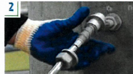
2 Remove the nut, the face washer and the spring shear sleeve and slide along the handle of the tool.
