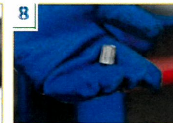
8 Press the small trigger on the shear wrench to eject the bolt spine. The application is now complete.
