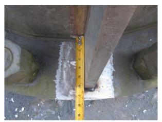
Installation of new stiffeners at the base plate.
