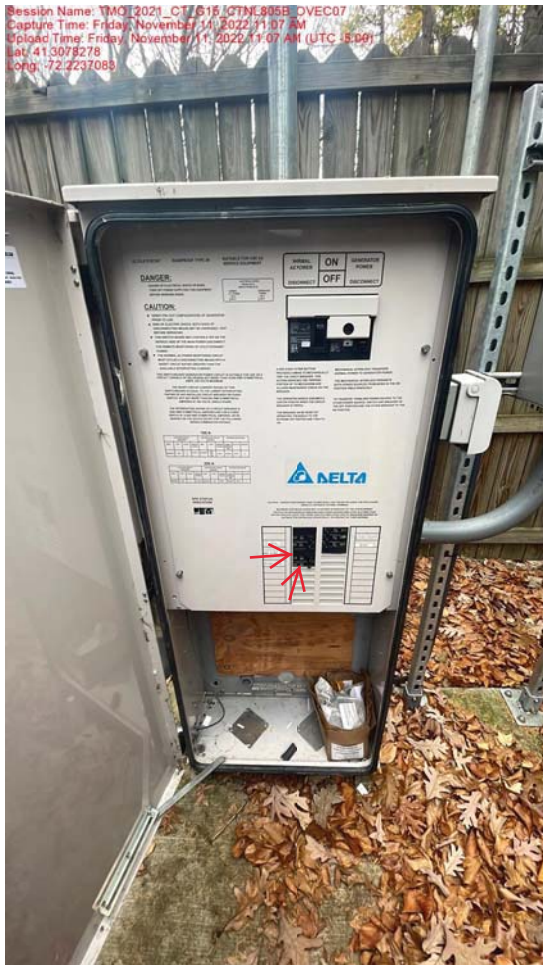
New Cabinets Tied Into Existing Electrical Cabinet
