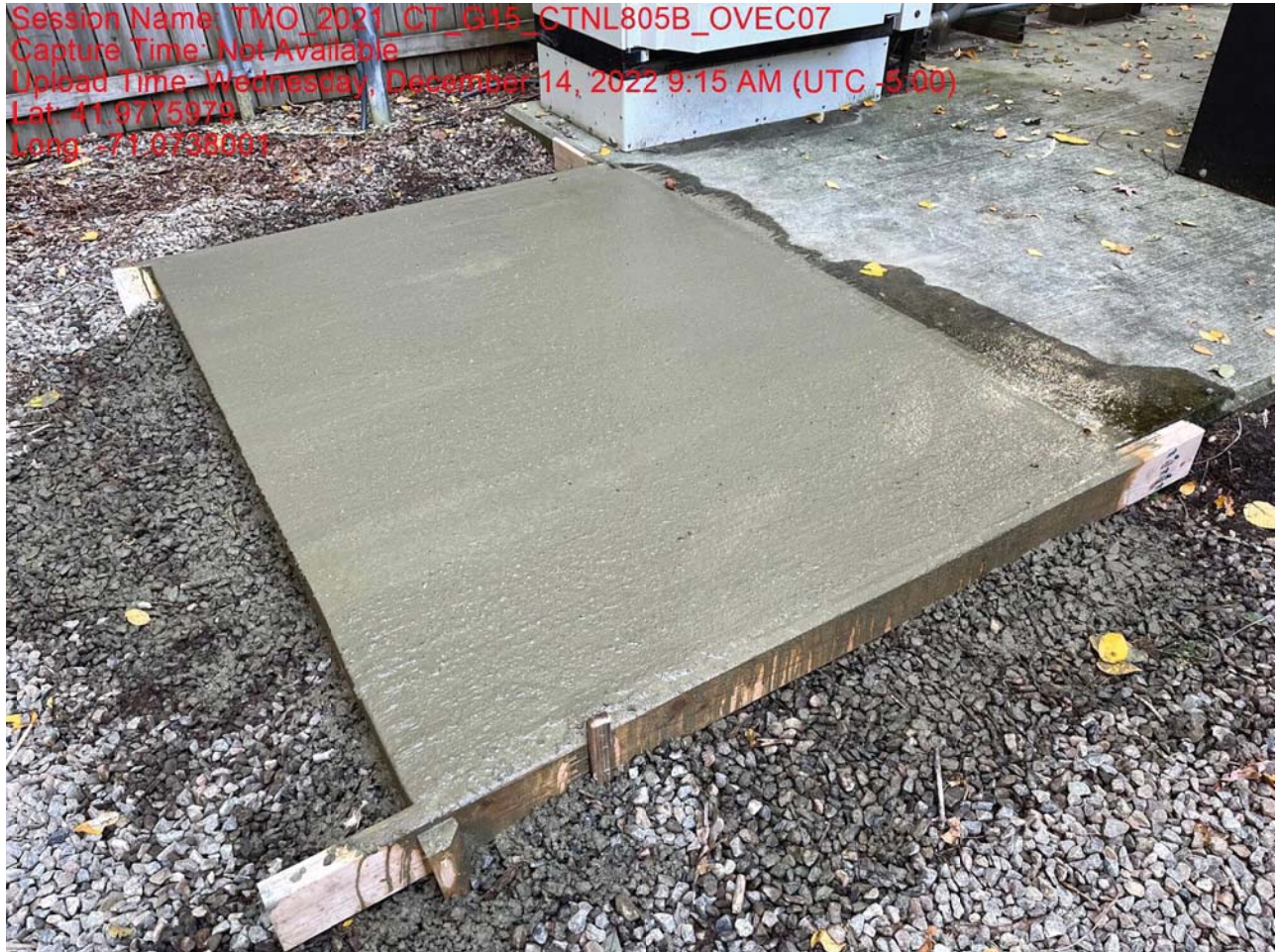
New 7'x5' Concrete Pad Extension
