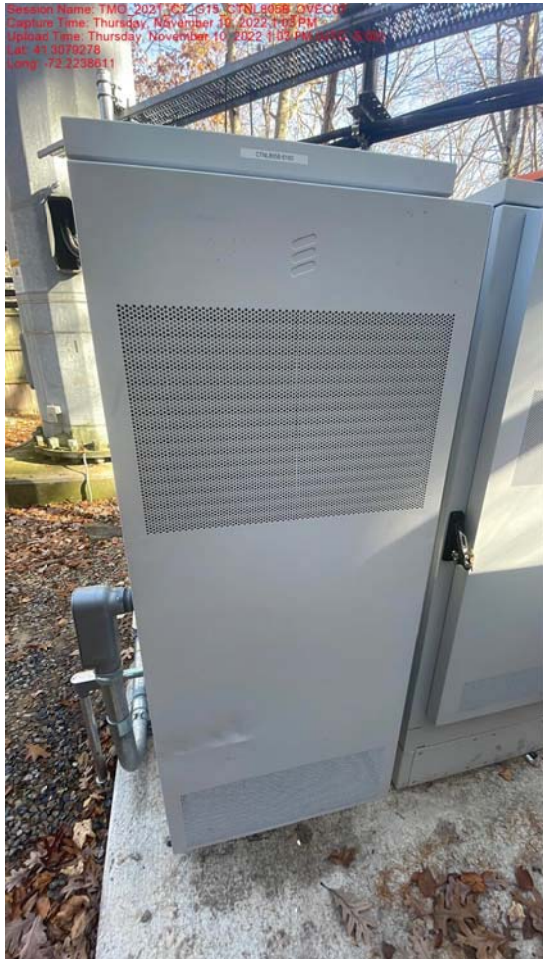
New Equipment Cabinet Mounted To Concrete Pad
