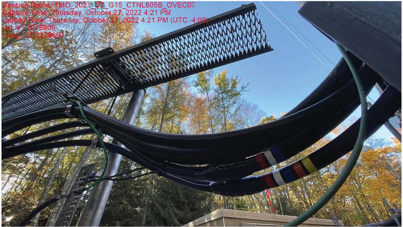
(1) New Signal Cable Run Along Existing Ice Bridge
