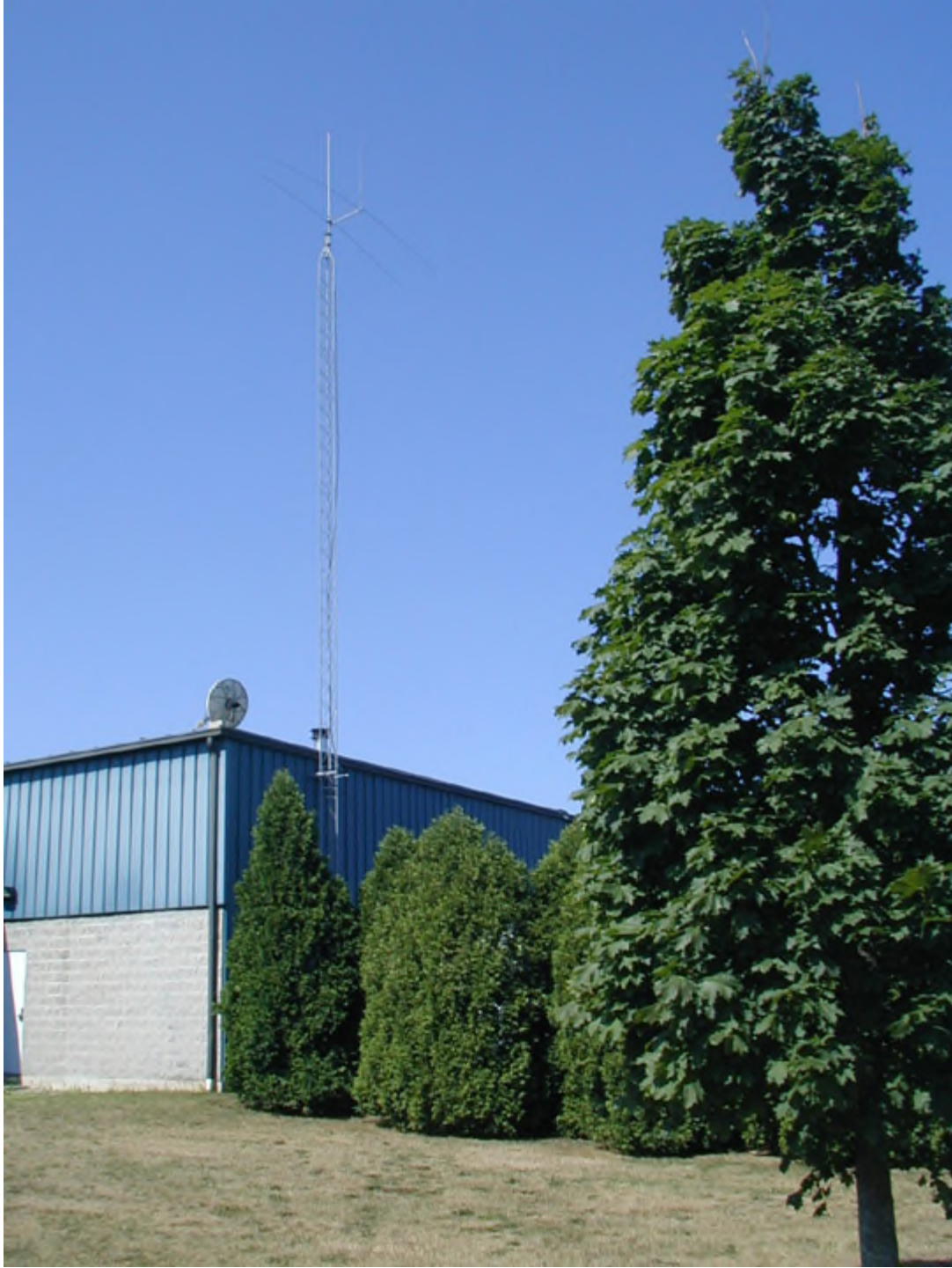
View of Back of Building Where Compound Will Be Located
