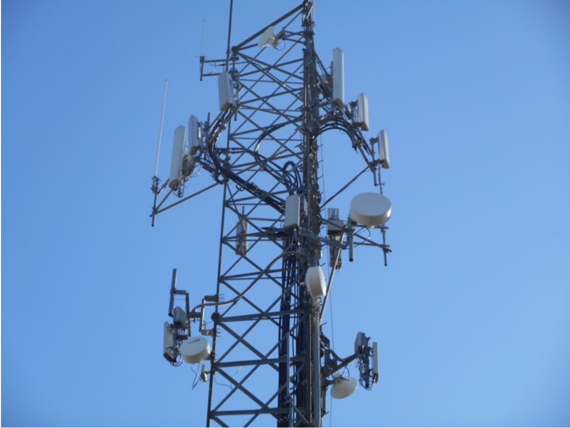
Photo 1: Photo illustrating the Tower with Appurtenances shown.
