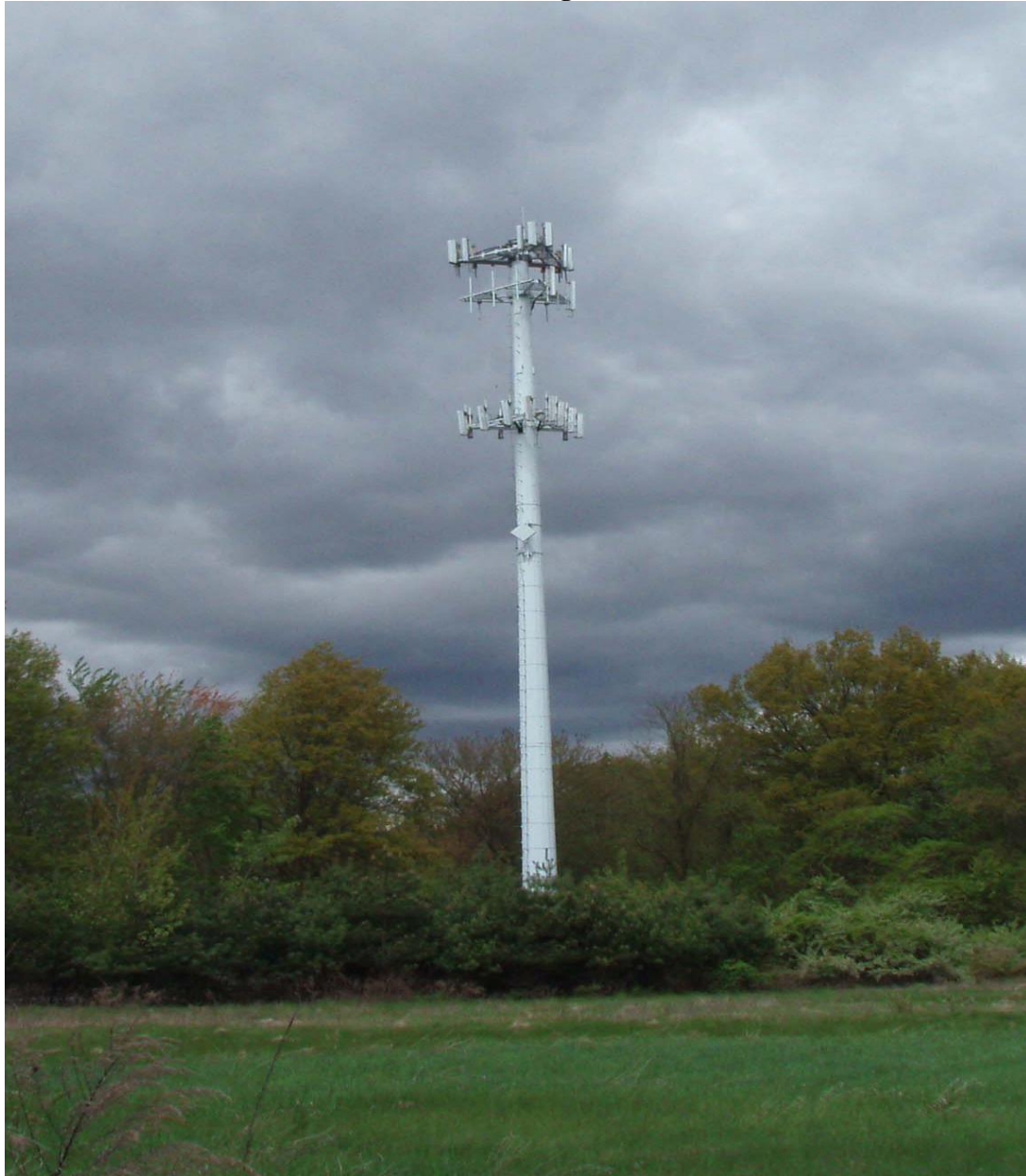
View of Existing Tower
