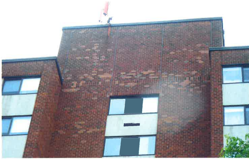
Photo 3: Sample photo illustrating the existing penthouse where the new sector C antennas are proposed to be located.
