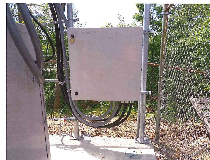
4 EXIST FIBER DISTRIBUTION BOX SCALE: NTS
