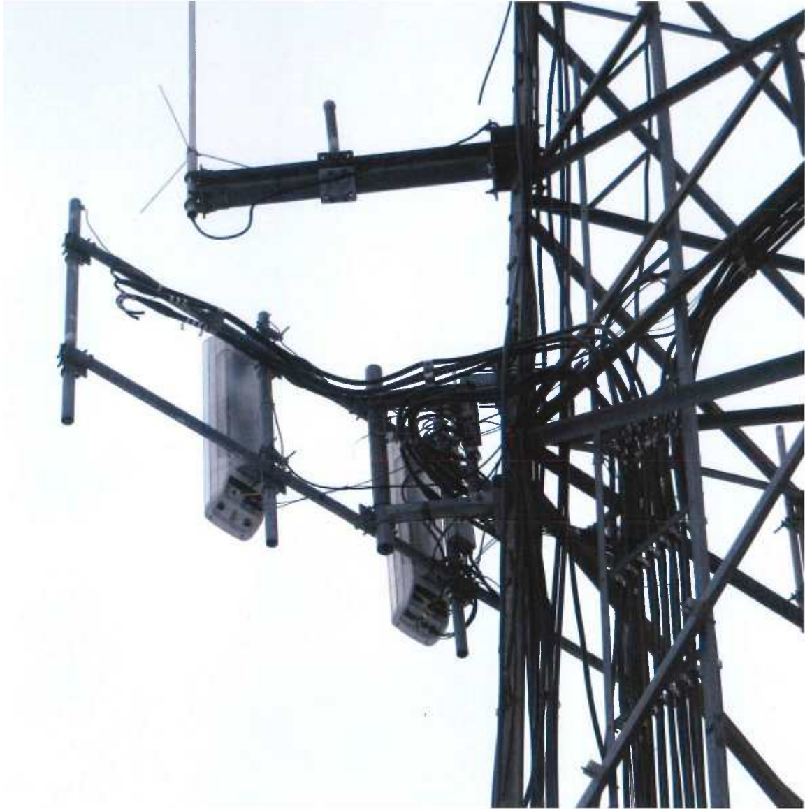
Photo 1: Photo illustrating the tower with Appurtenances shown.
