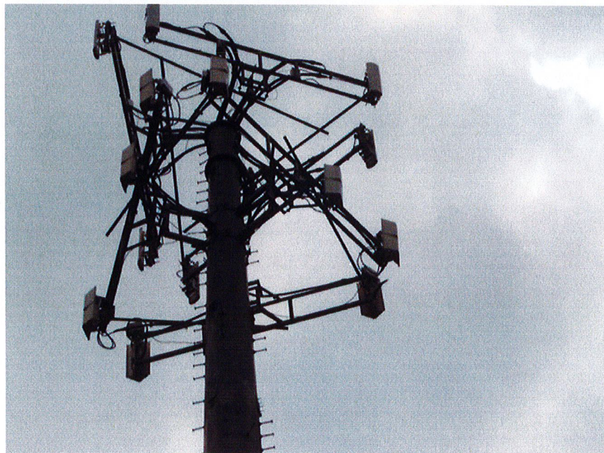
AT&T ARRAY REMOVED AT 165'
