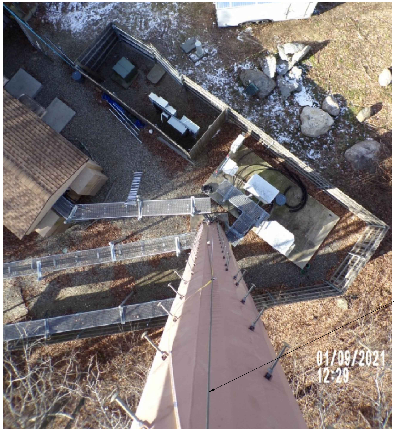
LOCATION OF SAFETY CLIMB
