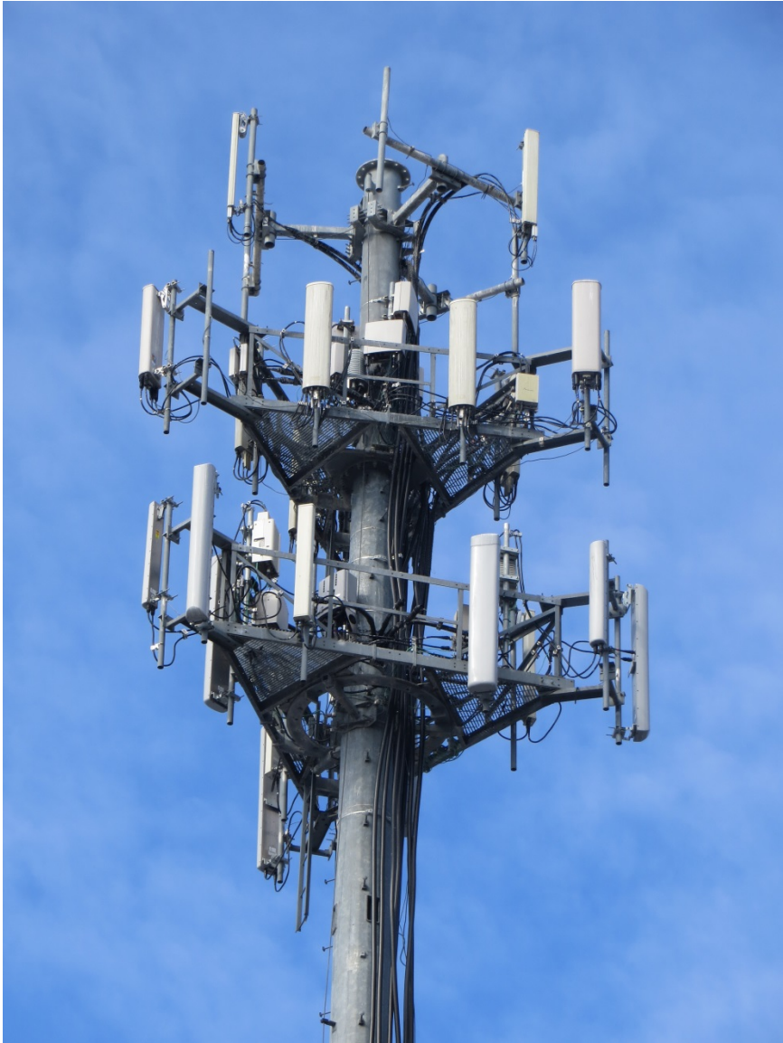
Photo 1: Photo illustrating the monopole with Appurtenances shown.
