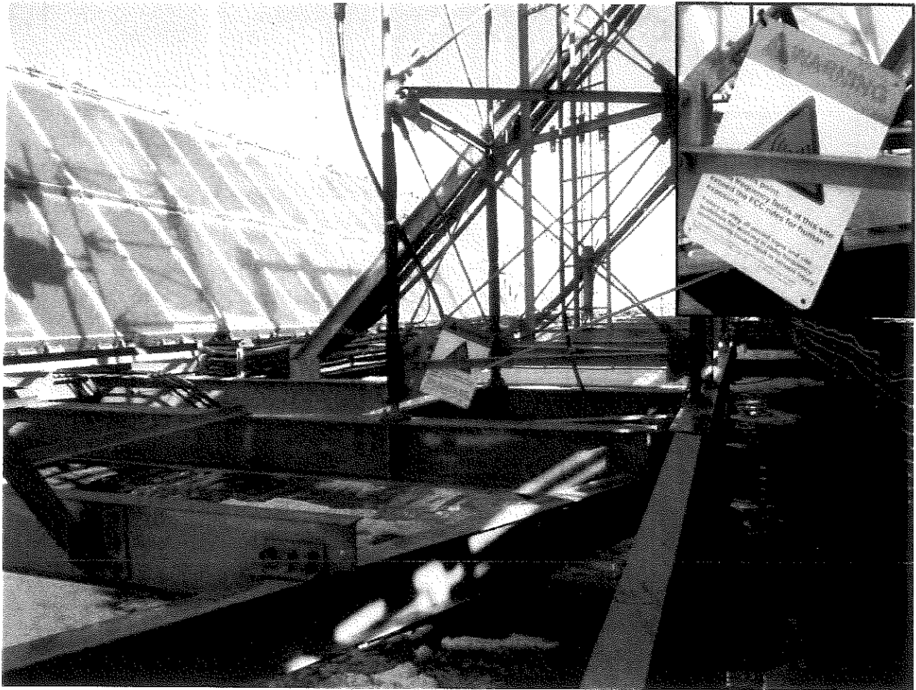
Figure 7: Posted Signage near Upper Rooftop Lattice Tower
