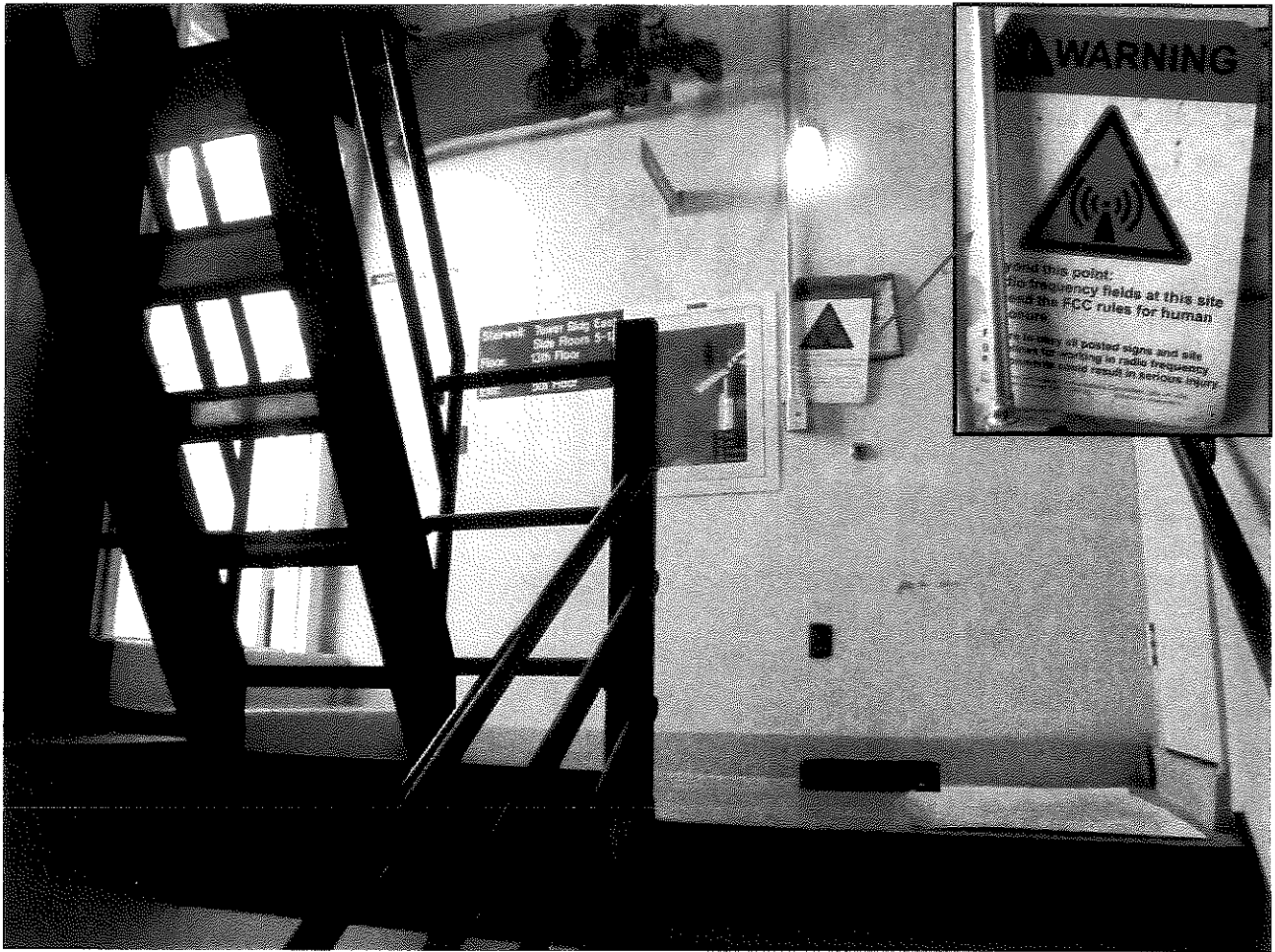
Figure 6: Posted Signage Near Eastern Lower Roof Access Points
