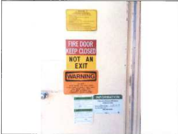
2. Signage on east roof access door
