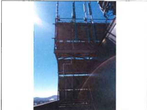
1. Verizon Sector B antennas
