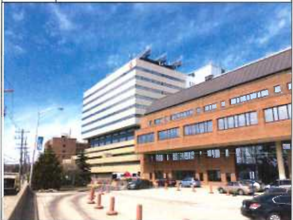
30. Site as viewed from ground
