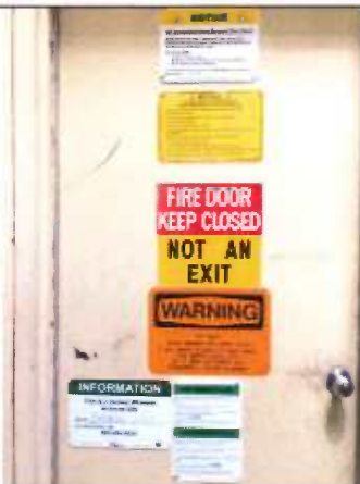
21. West roof access door signage
