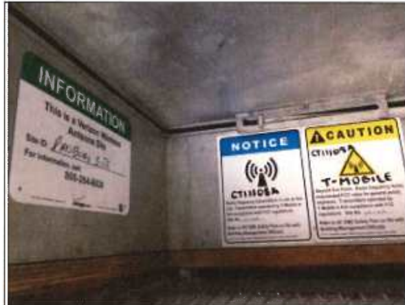
4. Signage on east upper roof access hatch
