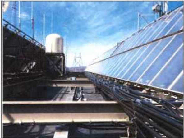
28. Upper roof looking east
