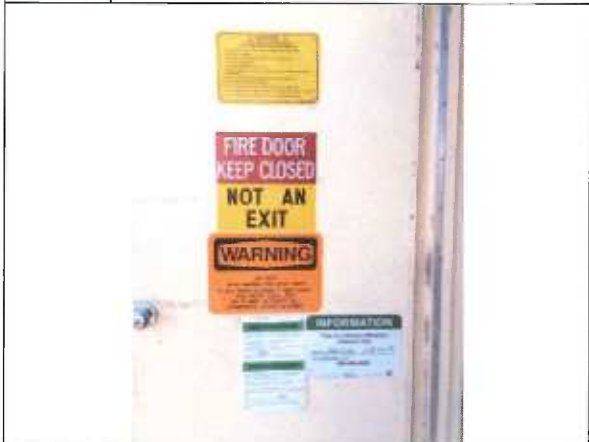
2. Signage on east roof access door
