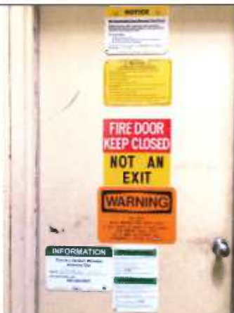
21. West roof access door signage
