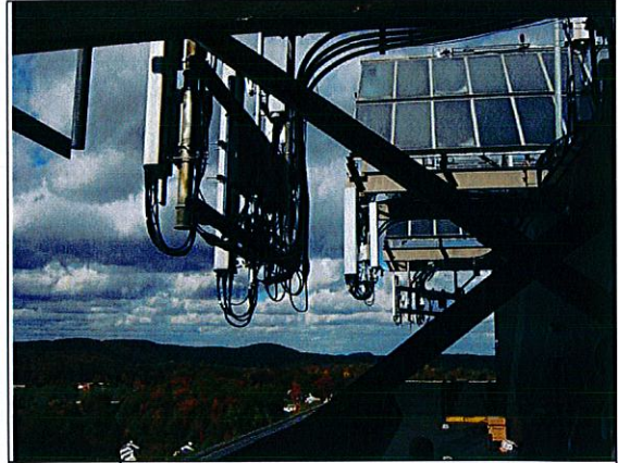
4. Nearest walking surface below AT&T and Sprint antennas
