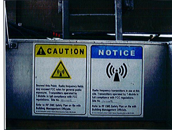
35. Signage on roof access hatch (typ.)
