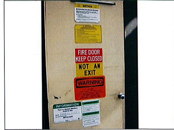
23. Signage on roof access door at top of stairwell B
