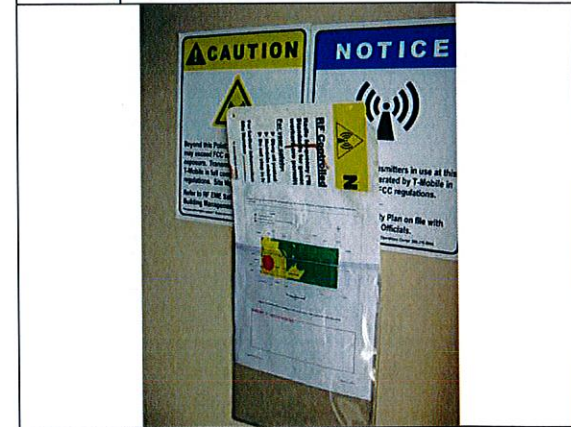
24. Signage beside roof access door at top of stairwell B
