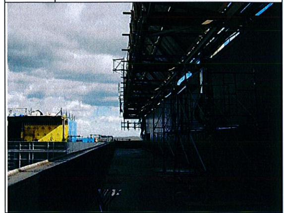
11. North roof overview looking east
