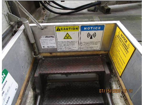
3. Access 2 with Existing Signage
