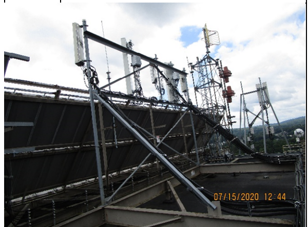
9. T-Mobile Sector B and D with Existing Signage
