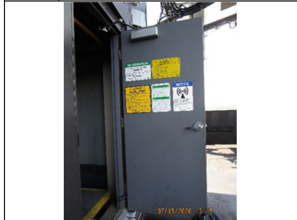
4. Access 3 with Existing Signage
