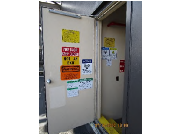
5. Access 4 with Existing Signage
