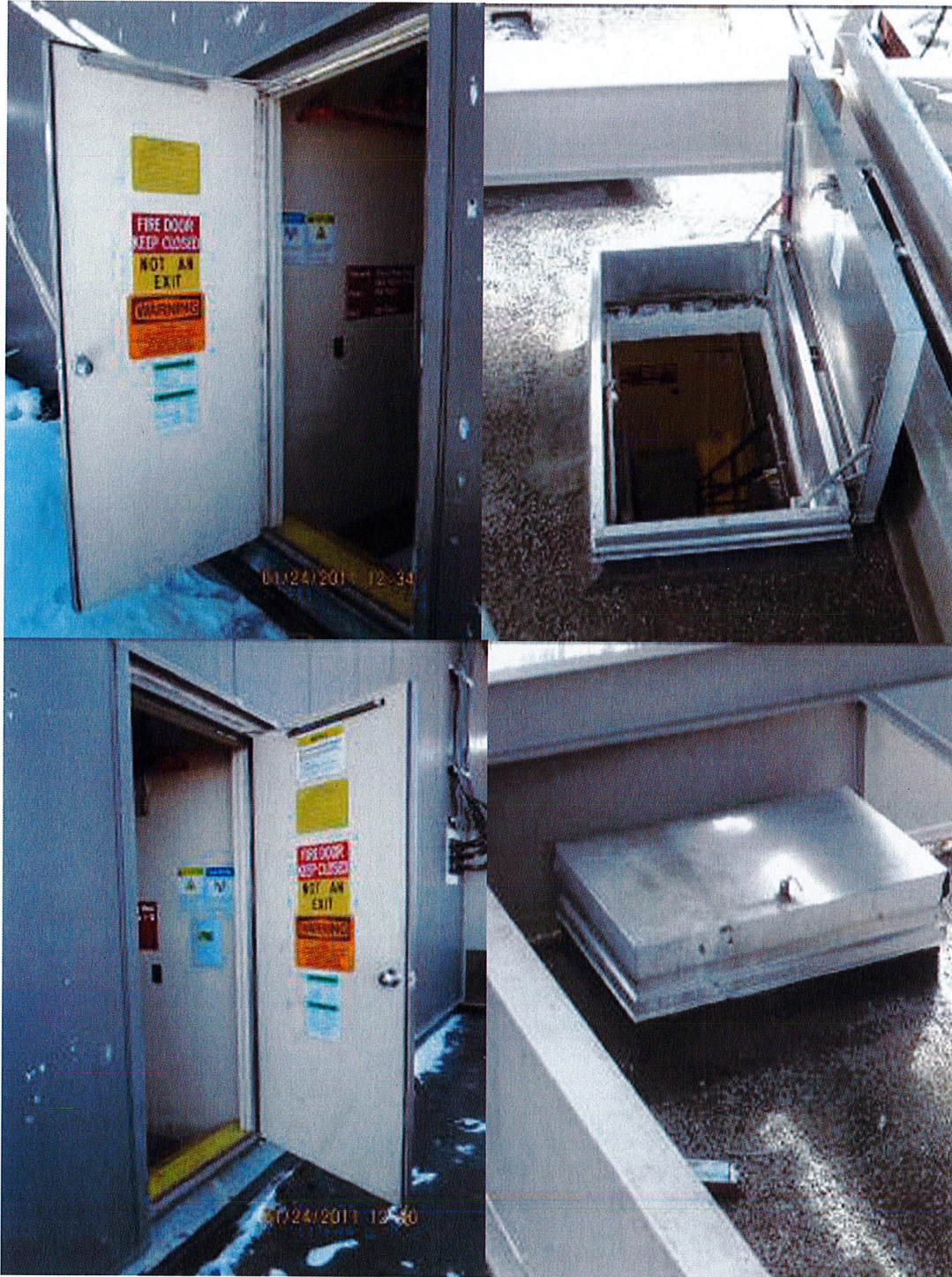
Figure 2: Roof Access Points & Posted Signage
