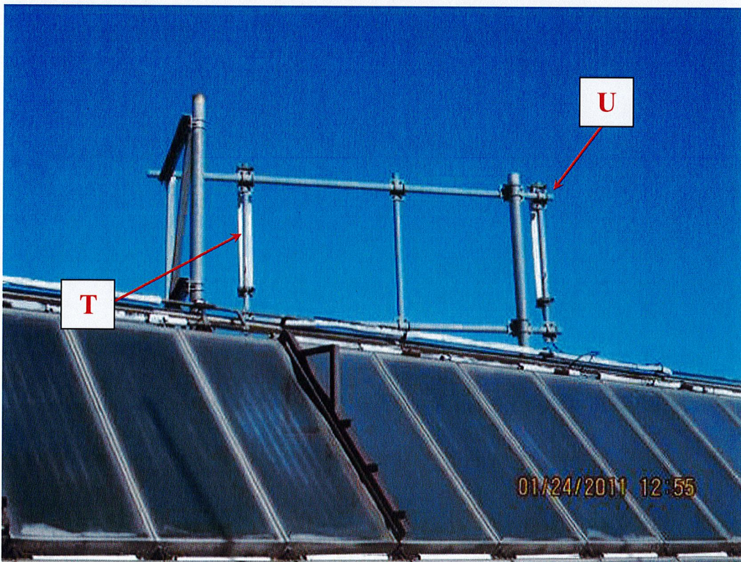
Figure 13: Antennas T & U (Sprint Alpha Sector)
