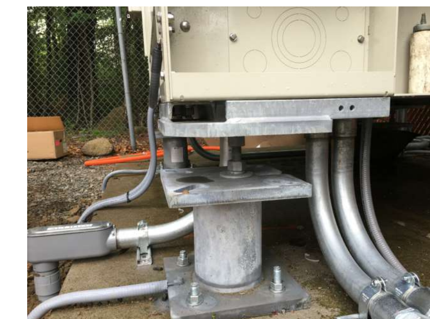
TYP. FOUNDATION WIC BASE ATTACHMENT KIT
