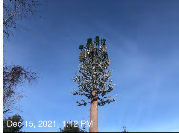
10. Existing T-Mobile and VZW Antennas – Sector C
