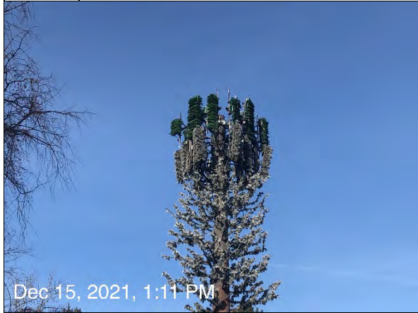
8. Existing T-Mobile and VZW Antennas – Sectors B and C
