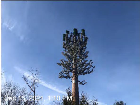
6. Existing T-Mobile and VZW Antennas – Sector B
