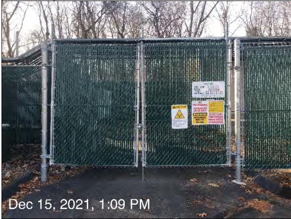
2. Locked Site Access Gate
