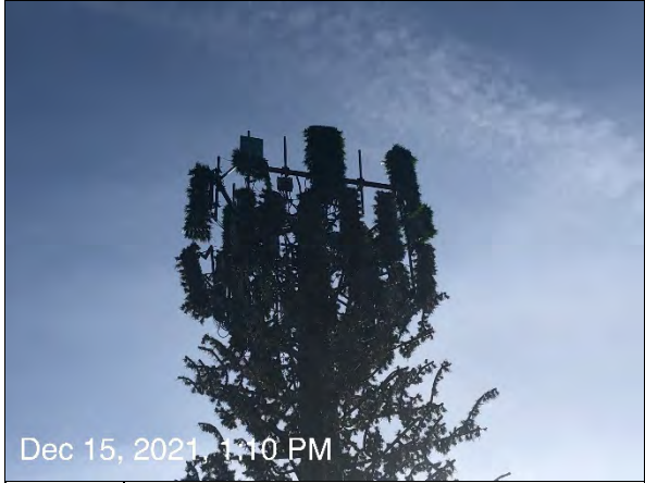
5. Existing T-Mobile and VZW Antennas – Sector A
