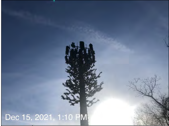
4. Existing T-Mobile and VZW Antennas – Sector A
