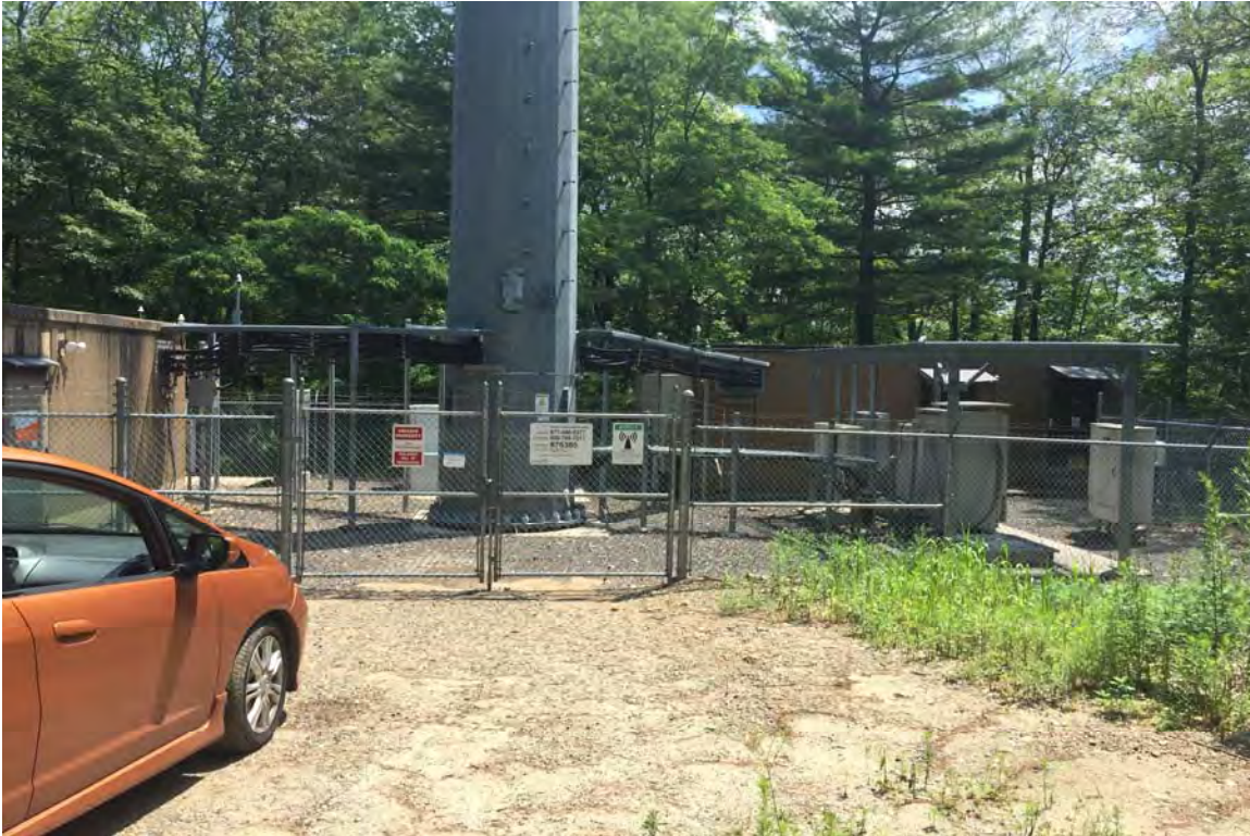
Photo 1: View of existing tower facility and compound, looking northeast.
