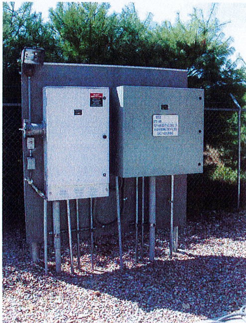
AT&T AC & TELEPHONE EQUIPMENT TO BE REMOVED
