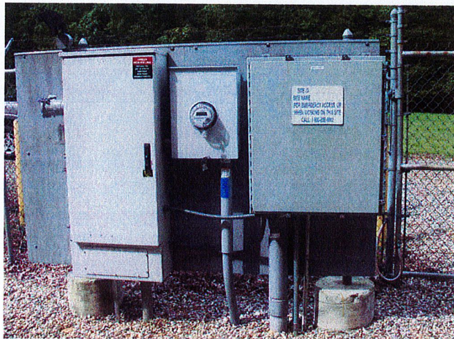
AT&T AC & TELEPHONE EQUIPMENT TO BE REMOVED
