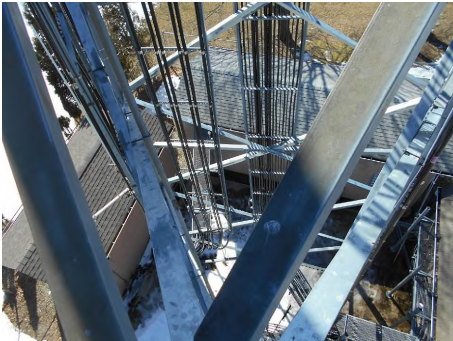
Photo of existing waveguide ladder.
