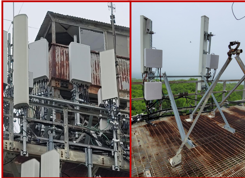
Figure 1 Existing Antenna Mount, Frontal view (left), Back view (back).
