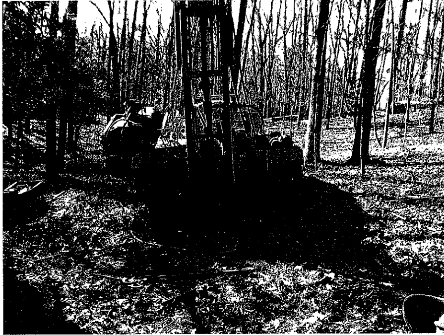
BEDROCK CORING AT PROPOSED TOWER FOUNDATION
